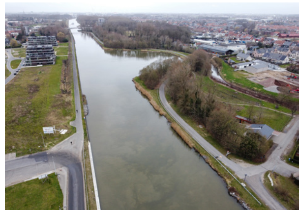
Location for the new bridge
