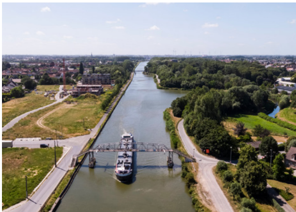
Former Lys Bridge in Ingelmunster
